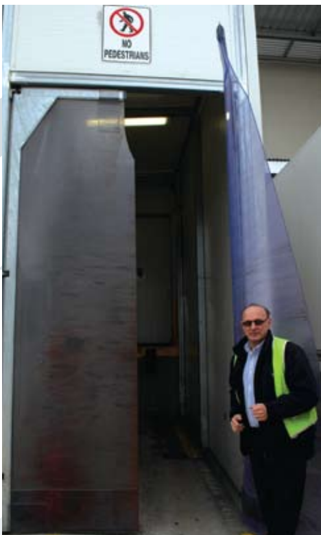
Air locks improve insulation and save energy
